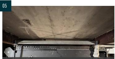
SCENE 5: And while the hard part MAY have seemed to be getting the hoist into the building, there was a special set of unique challenges getting it into position here where it had to navigate laterally between two beams with less than 2" of clearance on each side for a distance of FIFTEEN FEET from where it went up from the spot shown in Scene 3.
