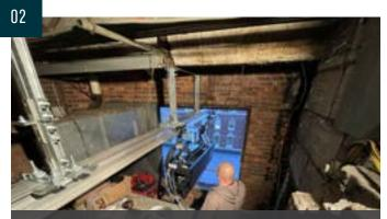
SCENE 2: Once we had the hoist up to the shaft opening, we were able to move it along the inside of the shaft using a custom temporary rail assembly and chain motors we rigged up that allowed us to ensure it could be moved safely and without coming into contact with other equipment.
