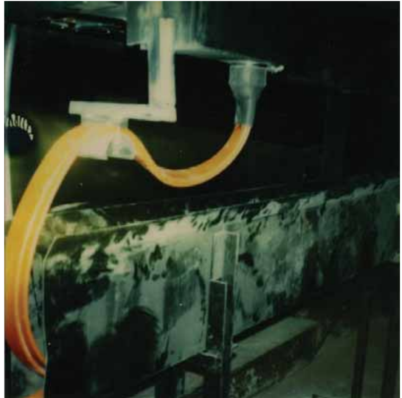
Figures 1 and 2 – MGM Reno side stage wagon showing cable trough arrangement
