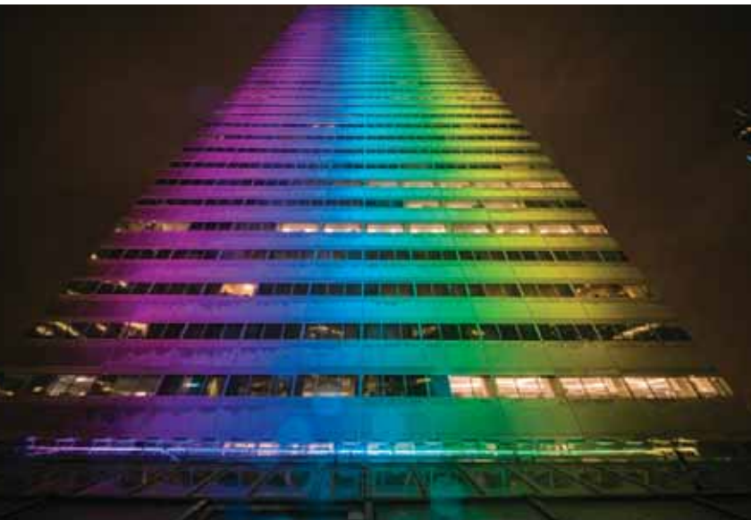
Façade lighting for One Financial Center in Boston, MA.
